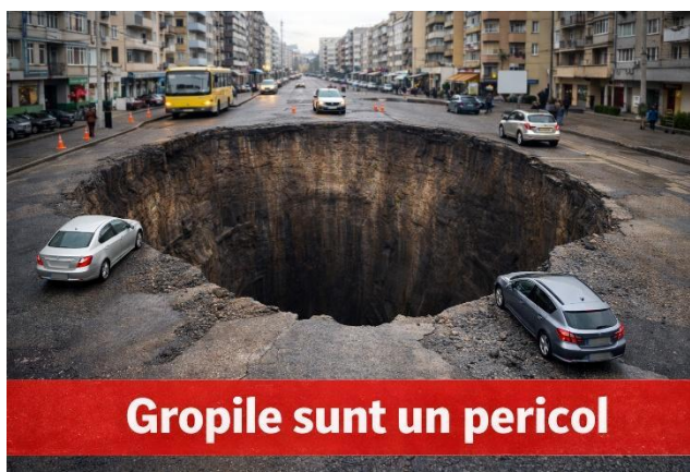
2. Cars almost fell into pothole; authorities to blame?
